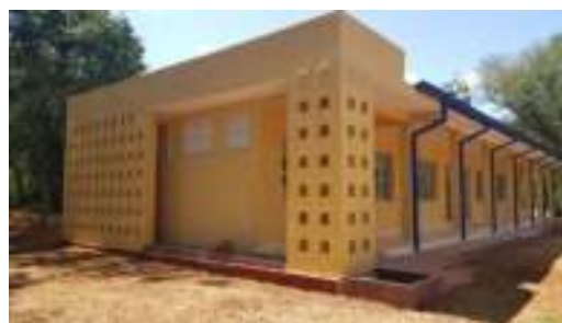
Ward Complex - District Ayurvedic Hospital Dehiyathakandiya, Ampara TCE : 11.00 mn Source of Fund : PSDG
