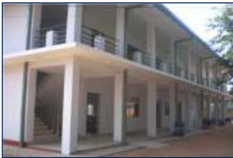
Emergency Treatment Unit - Santhively TCE : 12.50 mn Source of Fund : SHSDP
