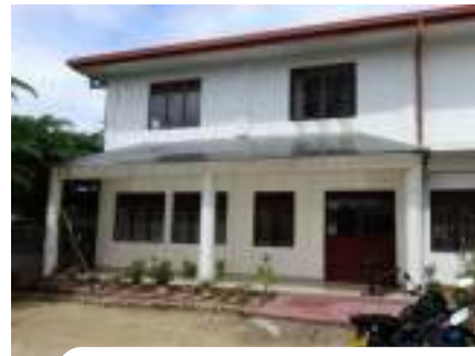
OPD Building - BH Eravur TCE : 23.90 mn Source of Fund : SHSDP
