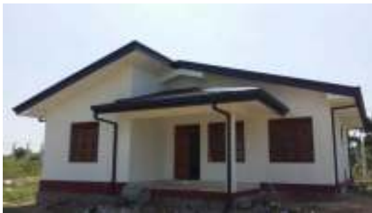
Garment Factory Quarters- Infrastructure Development, Seethanaveli, Muthur TCE : 10.00 mn Source of Fund : BRD
