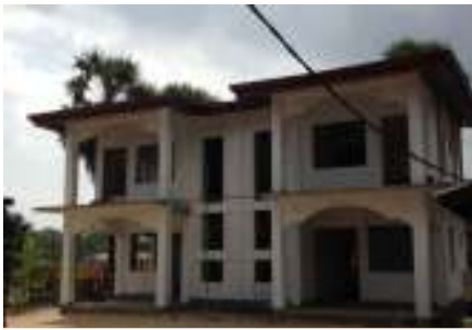
Consultant Quarters at Base Hospital Kaluwanchikudy TCE : 10.80 mn Source of Fund : PSDG
