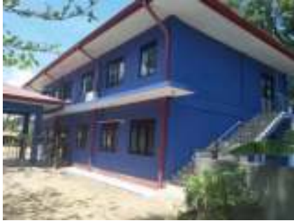
Laboratory and Drug Store - BH, Valaichchenai TCE : 20 mn Source of Fund : SHSDP
