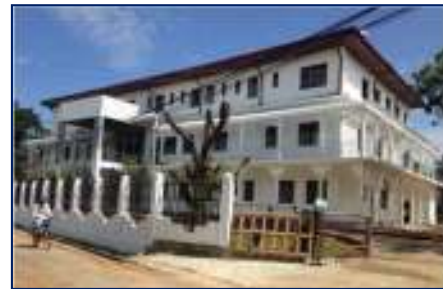
Base Hospital Kaluwanchchikudy - Batticaloa TCE : 300 Mn Source of Fund : JICA
