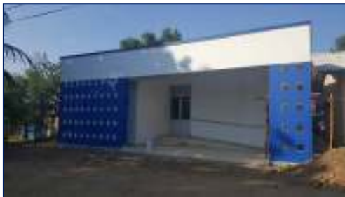
Periodic Ward Complex - Central Camp, Ampara TCE : 8.00 mn Source of Fund : SHSDP
