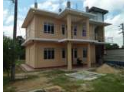
Nursing officer's Quarters - Valaichchenai TCE : 4.70 mn Source of Fund : PSDG
